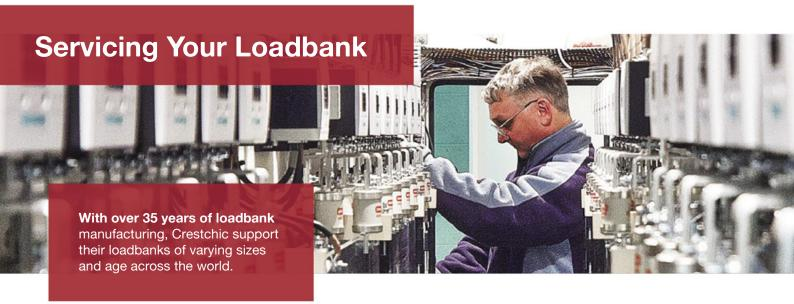
A Crestchic service visit helps keep your loadbank in peak condition with regular maintenance and software upgrade visits scheduled at your convenience. Our data module calibration service ensures that the applied electrical load is accurate over a 12 month period, with traceability to UKAS laboratory standards.
